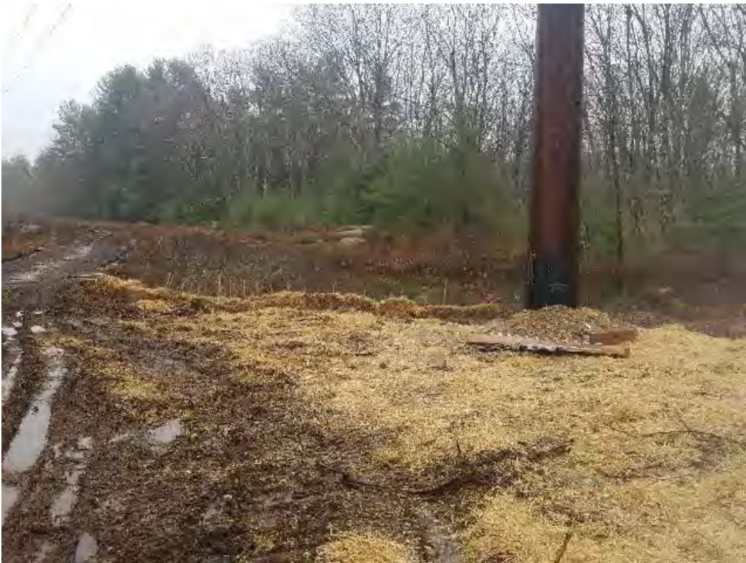
Fig 14: Str. 80 work area. Viewing southeast. (05-01-20).
