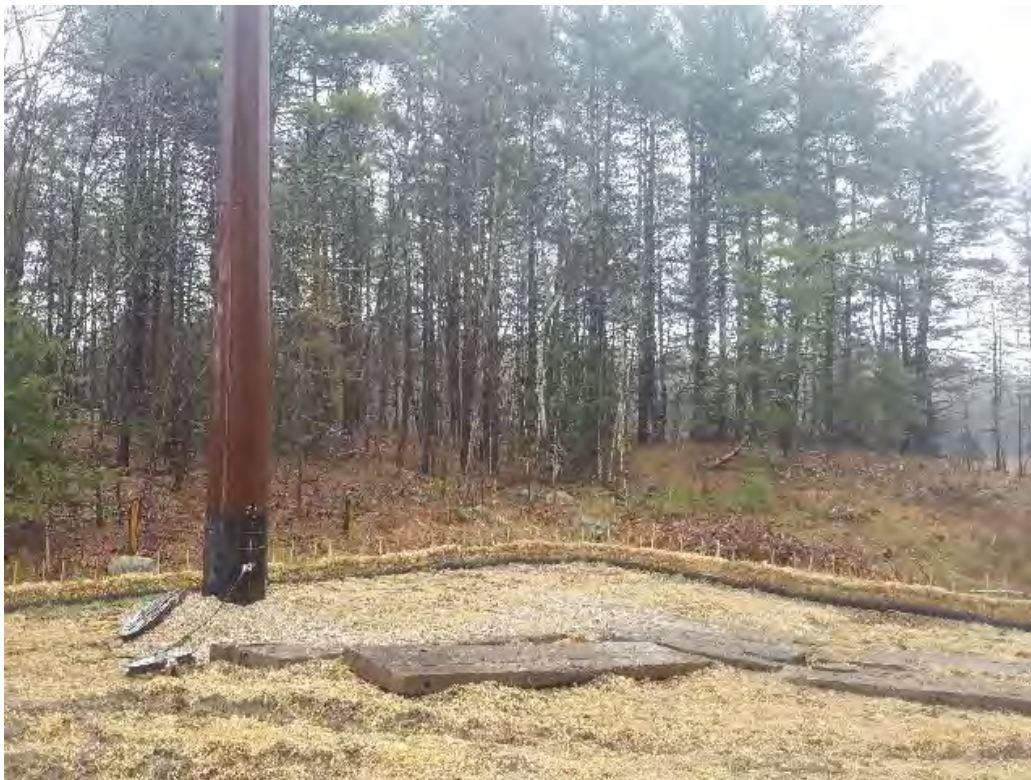
Fig 10: Str. 93 work area. Viewing east. (05-01-20).
