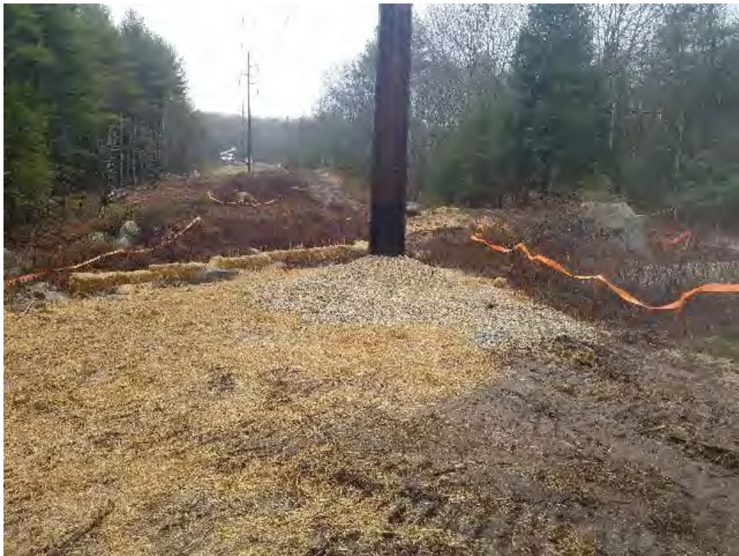
Fig 6: Str. 83 pole set and work area. Viewing east. (05-01-20).
