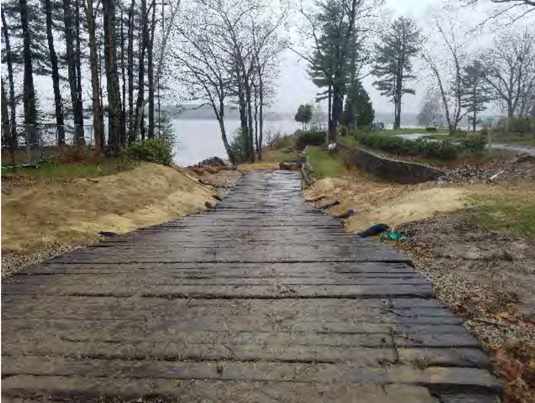
Fig 1: Timber mat access road to intertidal zone at Gundalow landing/east side of the Bay. Viewing southwest. (05-01-20).
