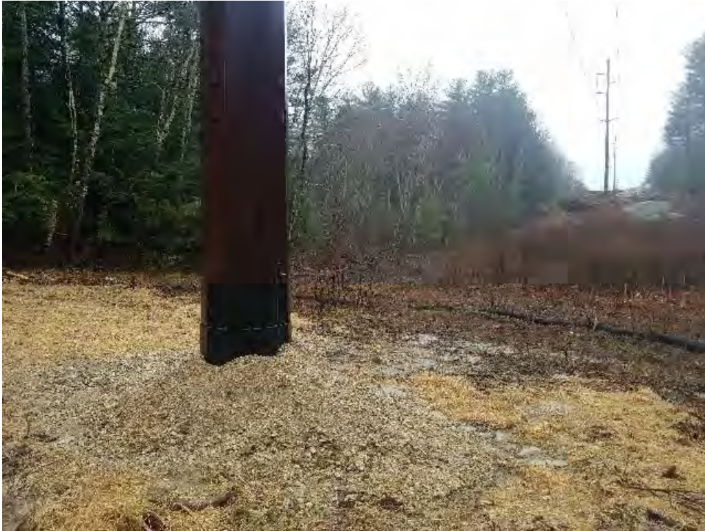
Fig 7: Str. 82 pole and work area. Viewing west. (05-01-20).
