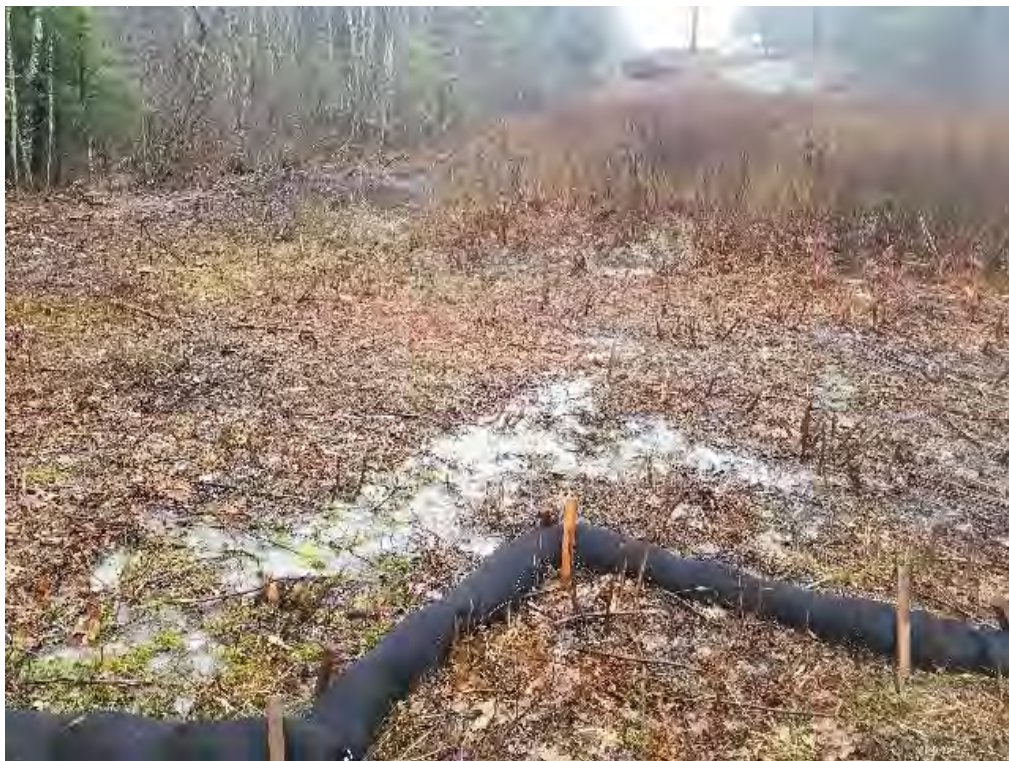
Fig 8: Minor turbid water flowing into wetland DW38; downslope of Str. 82. Viewing west. (05-01-20).
