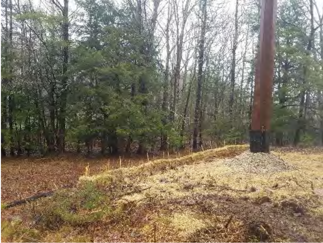
Fig 11: Str. 91 pole and work area. Viewing northeast. (05-01-20).
