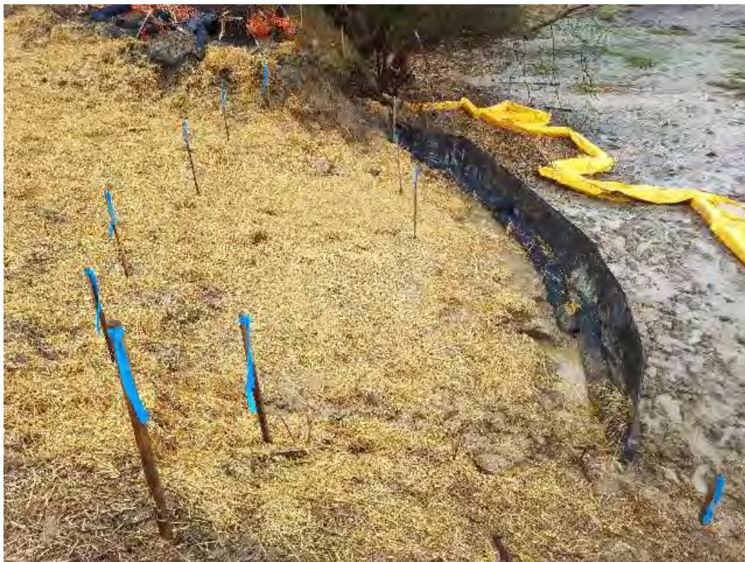
Fig 2: BMPs and exposed soils mulched at toe-of-slope at Gundalow landing/east side of the Bay. Viewing south. (05-01-20).
